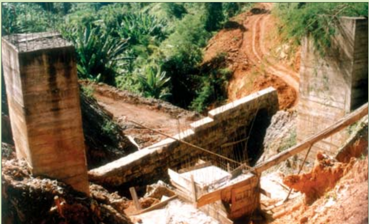
Construction of the Mali Hydro-electric power plant is far from complete; November 2004
