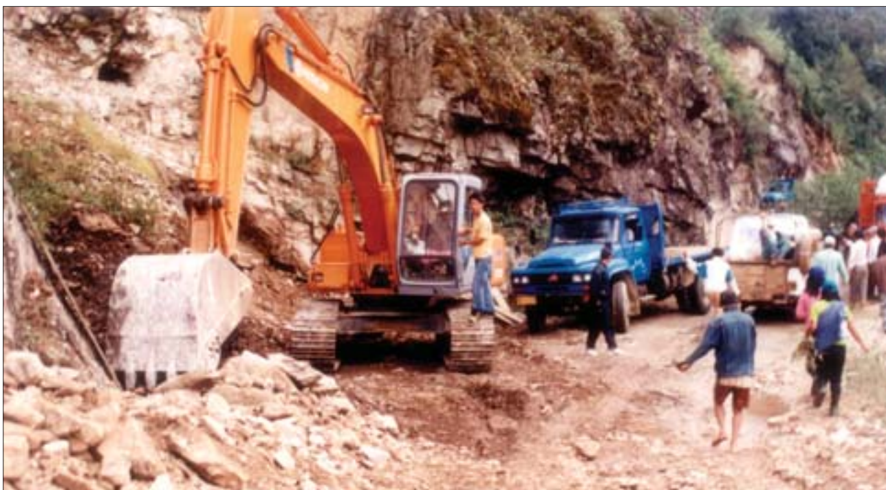
Chinese road construction in Kachin State (between Chipwe and Pangwah); 2004
